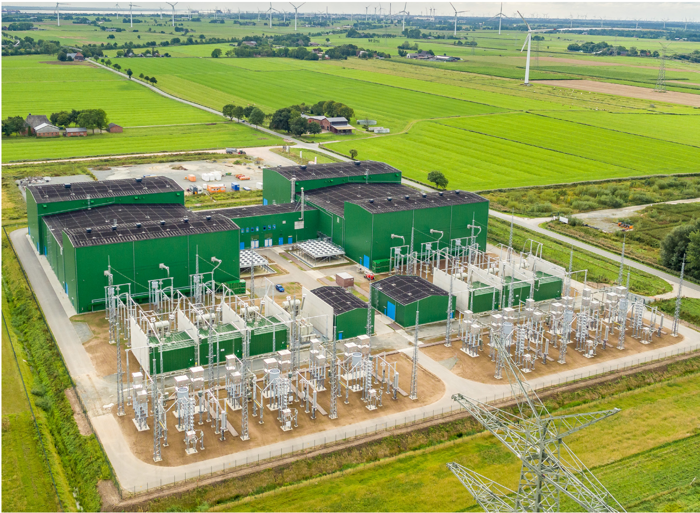
The NordLink converter station site in Wilster, Germany Source: TenneT
