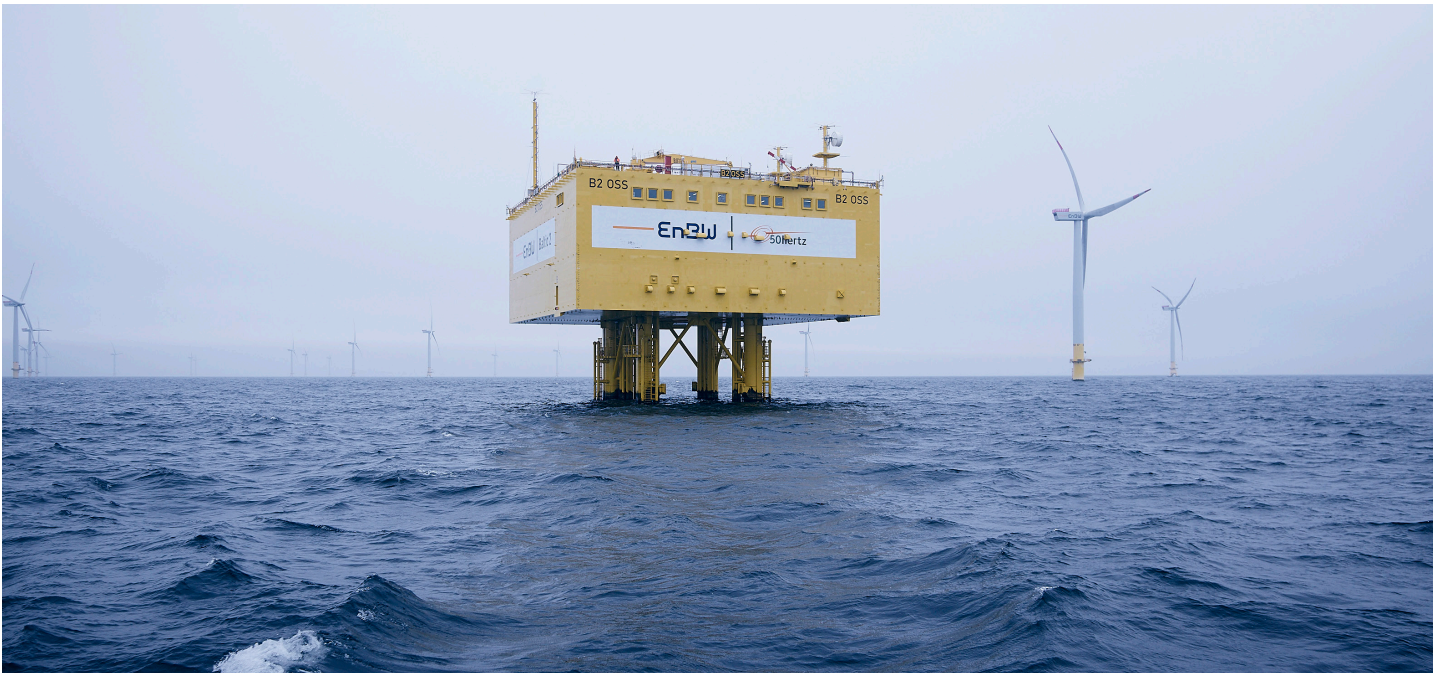
Combined Grid Solution and Bentwisch Converter Station Source: 50Hertz
