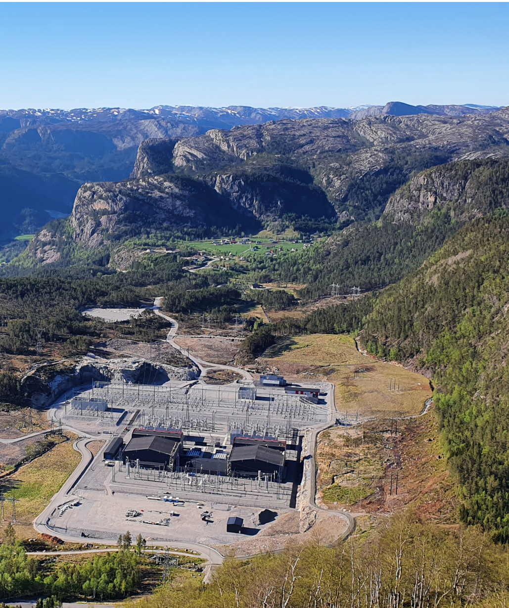
The completed NordLink converter station in Tonstad, Norway Source: TenneT
