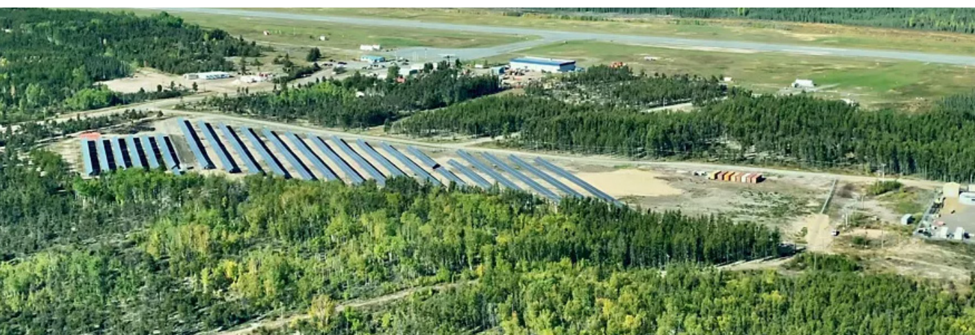
Aerial view of Fort Chipewyan microgrid site near Lake Athabasca, Alberta's oldest established community Source: 3NE
