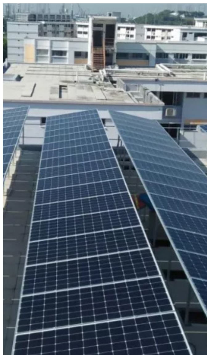
Solar photovoltaic (PV) systems on the rooftops of public housing. Photo credit: Housing Development Board (HDB)
