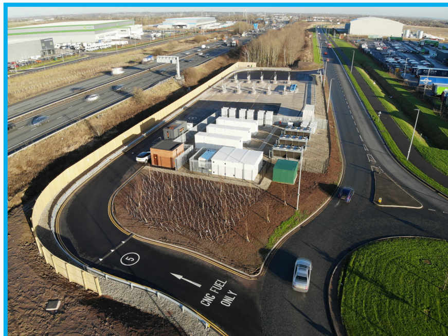
This station is located next to the M62, one of the busiest motorways in the UK, and is in the middle of a large logistics park, where more than 500 HGVs operate from daily.
